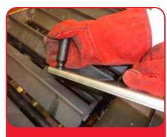
Step 7 - use the other end of the scraper to remove burnt-on debris from the pyramid radiants
